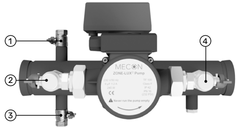
Fig. 8: Overview of main pipe commissioning
